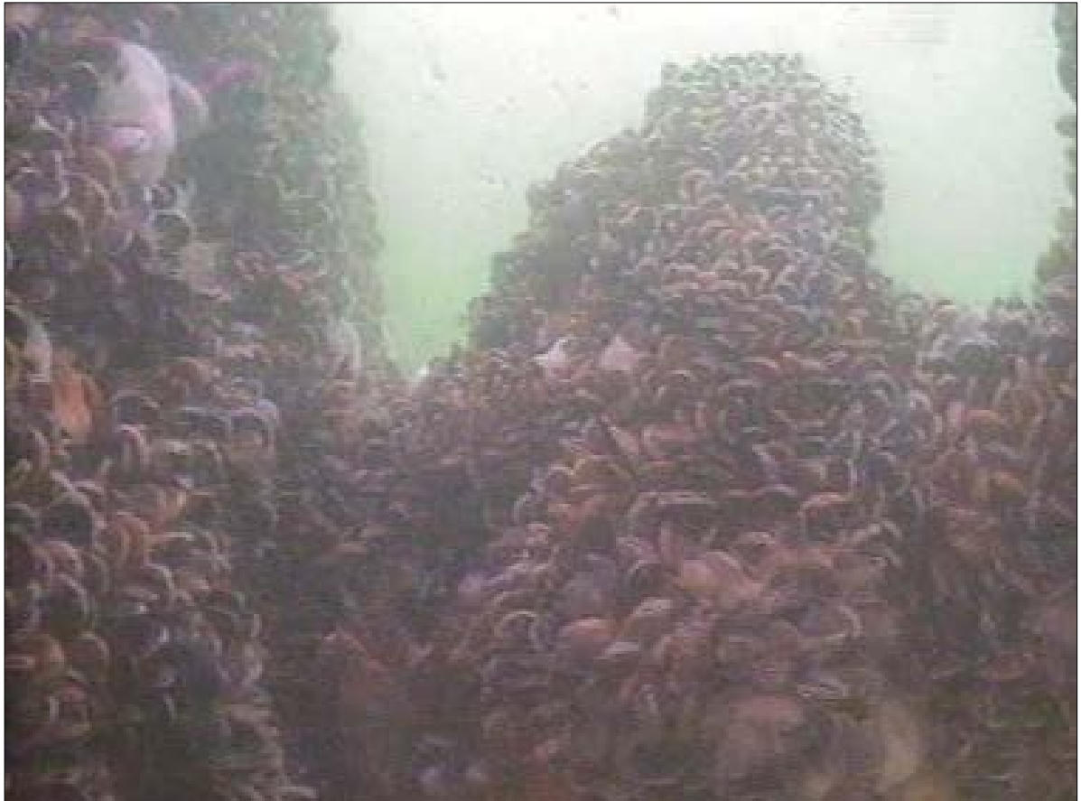
Figure 5.1: Dense mussels ( Mytilus edulis ) with Plumose anemone ( Metridium senile ) attached to a turbine foundation at the Barrow Offshore Wind Farm
