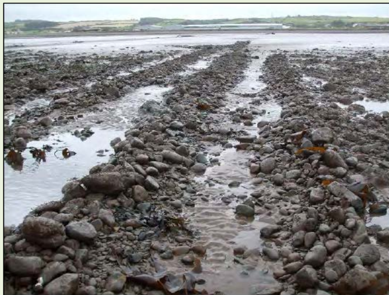
Figure 5.4: Physical impacts of export cable installation on the lower shore at Robin Rigg Offshore Wind Farm (source: Entec, 2009b)
