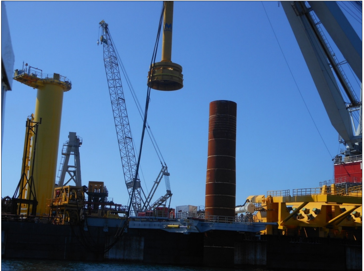
Figure 4.1: Hammer piling of a monopile
