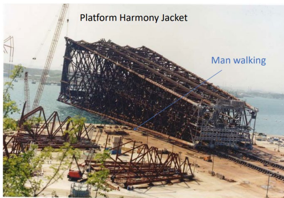
FIGURE 2-1 Platform Harmony Jacket Being Readied for Installation (Photo credit: ExxonMobil).
