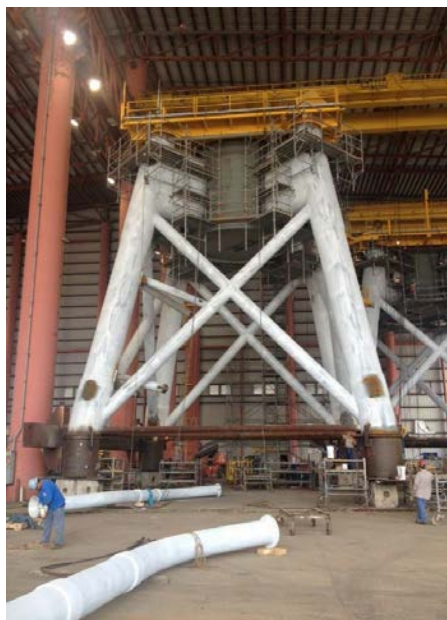
Fabrication of Block Island Foundations by Gulf Island Fabricators, in Houma, LA
