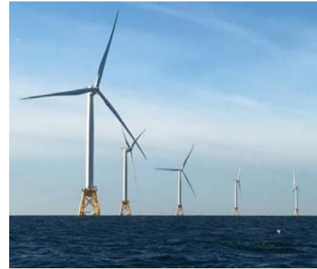
Block Island Wind Farm offshore Rhode Island
